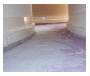
Goldfields Protective Coatings (GPC) was engaged by Evolution Mining for the refurbishment of their Carbon In-Leach (CIL) gold processing tank ring beams at their Westonia operations.
